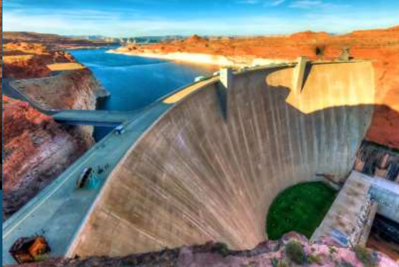
Decreases Risk of Losing Power Production at Glen Canyon Dam
