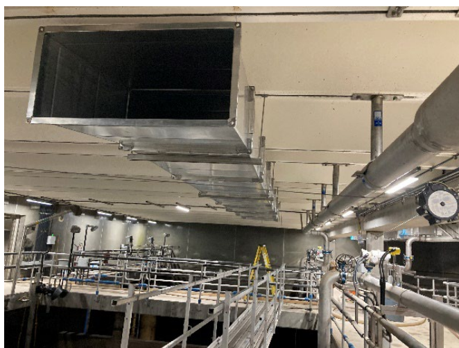
Duct installation over Aeration Basin 2
