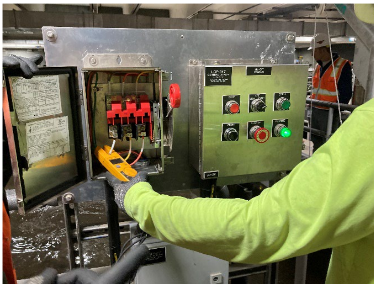
Startup and testing of Aeration Basin Mixing System, Zone 2G
