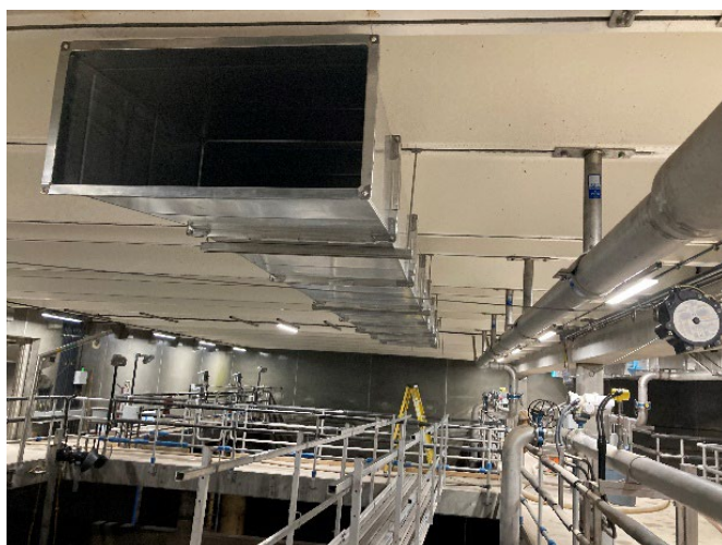
Duct installation over Aeration Basin 2
