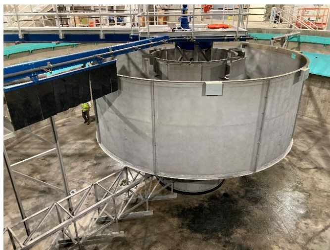
New Secondary Clarifier dewatered for inspection (SC-1)
