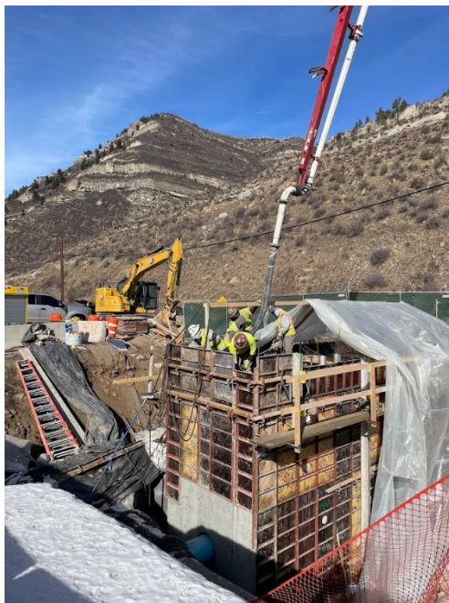
Placing concrete for the wet well lid
