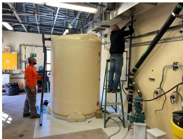
Sodium Hypochlorite Storage Tank Replacement at the Berry Creek Wellhouse
