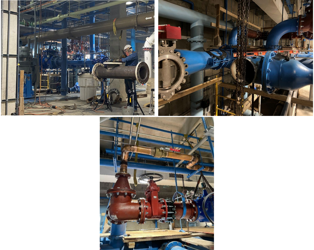
Pipe Fitting Work at the Avon Drinking Water Facility
