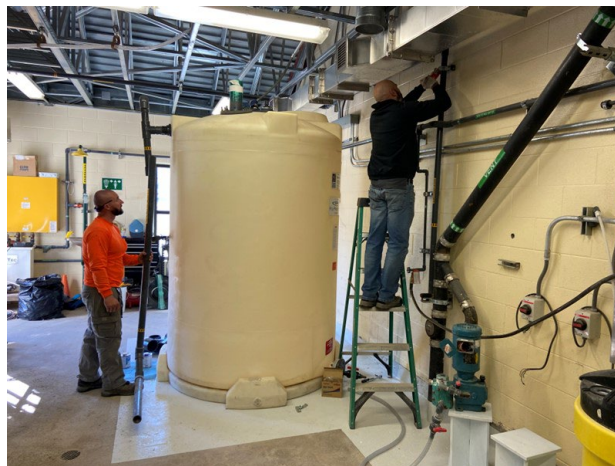
Sodium Hypochlorite Storage Tank Replacement at the Berry Creek Wellhouse
