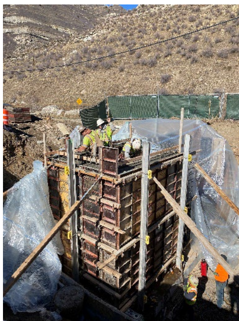
Placing concrete for the wet well wall
