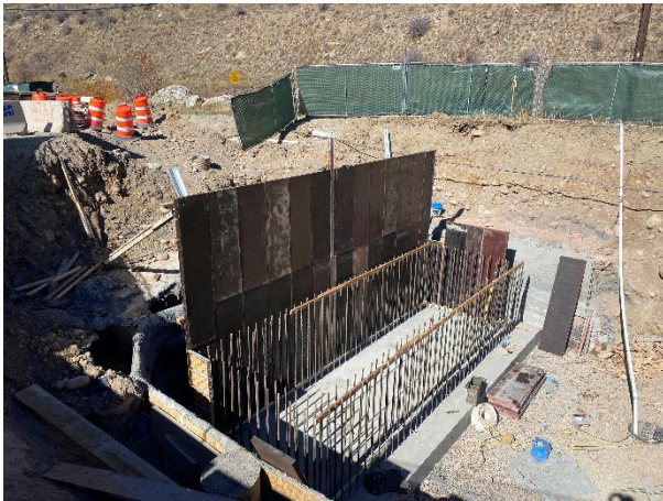
Setting forms for the wet well walls
