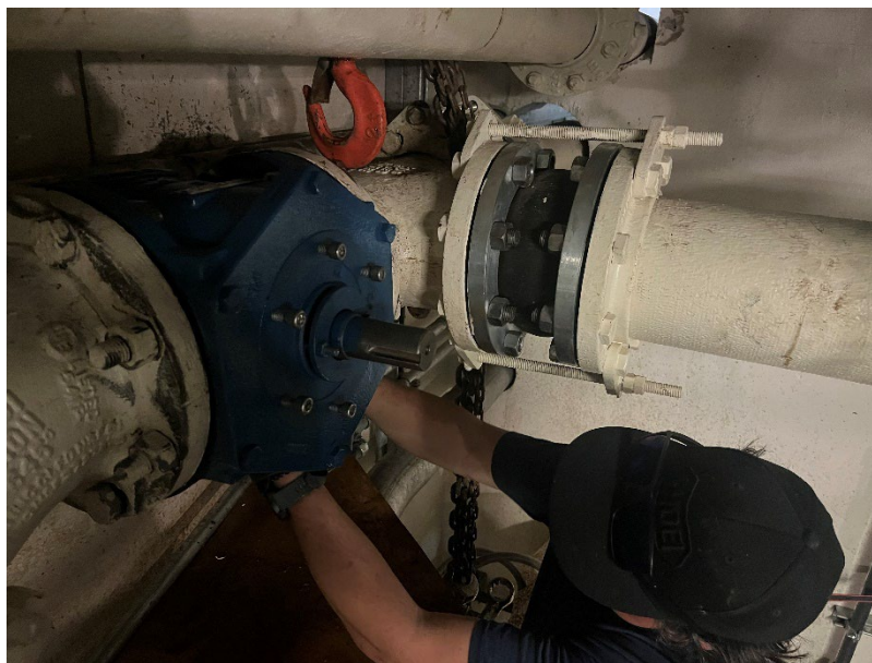
EWV Staff replacing critical ATAD transfer valve.
