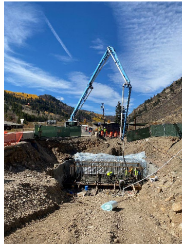
Gould placing concrete for the wet well slab on grade
