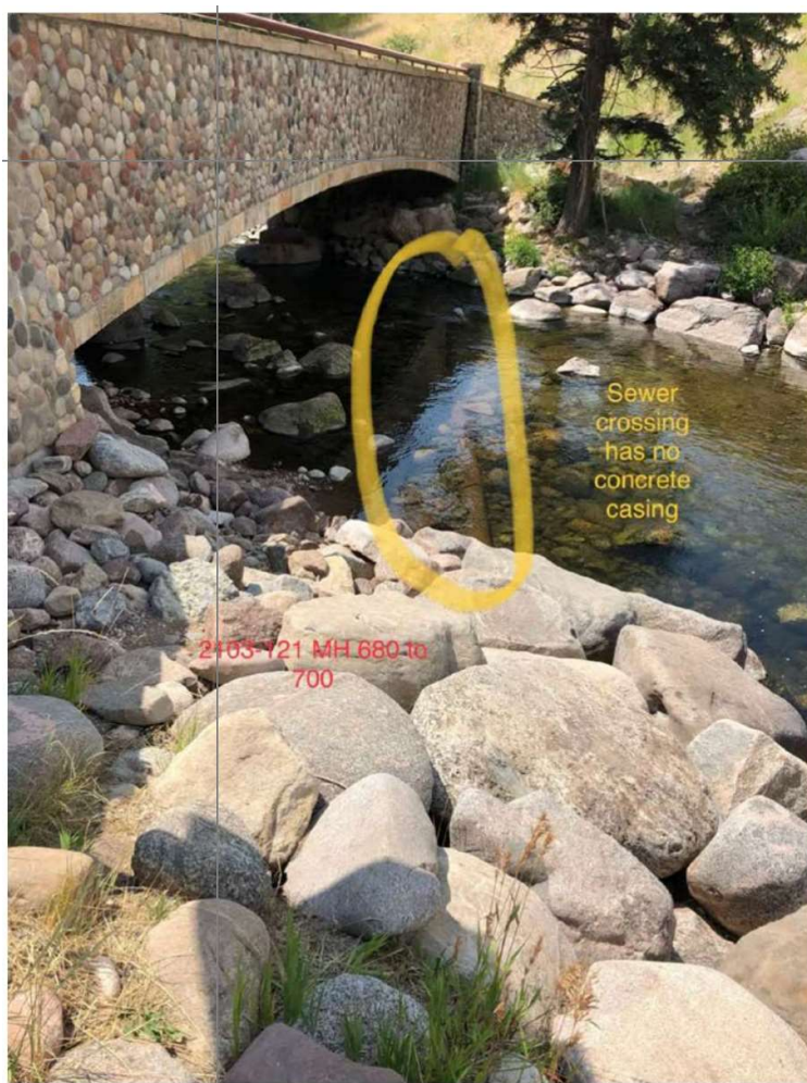
Figure 6: Sewer pipe without concrete casing
