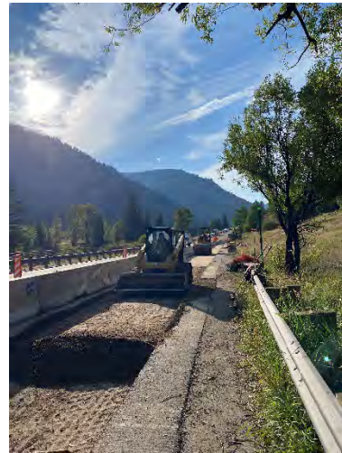
Gould backfilling and compacting in preparation for paving.
