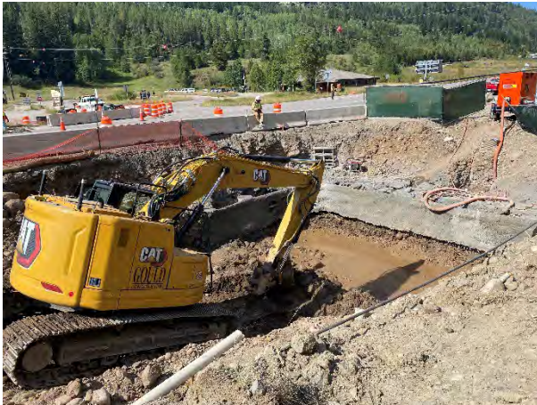
Excavation during shoring installation for the wet well.
