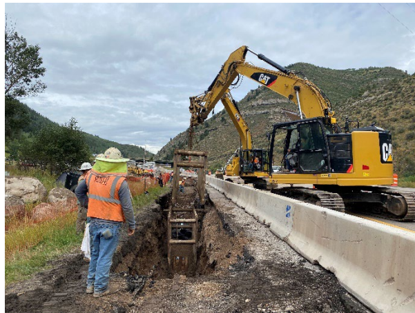
Gravity sewer line construction
