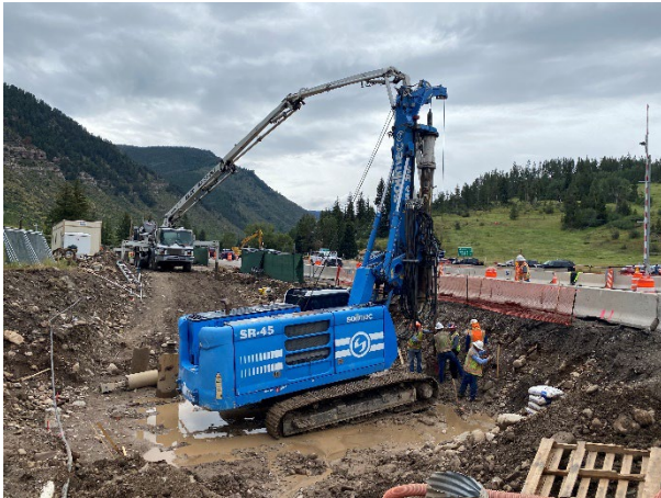
Drilling for wet well shoring
