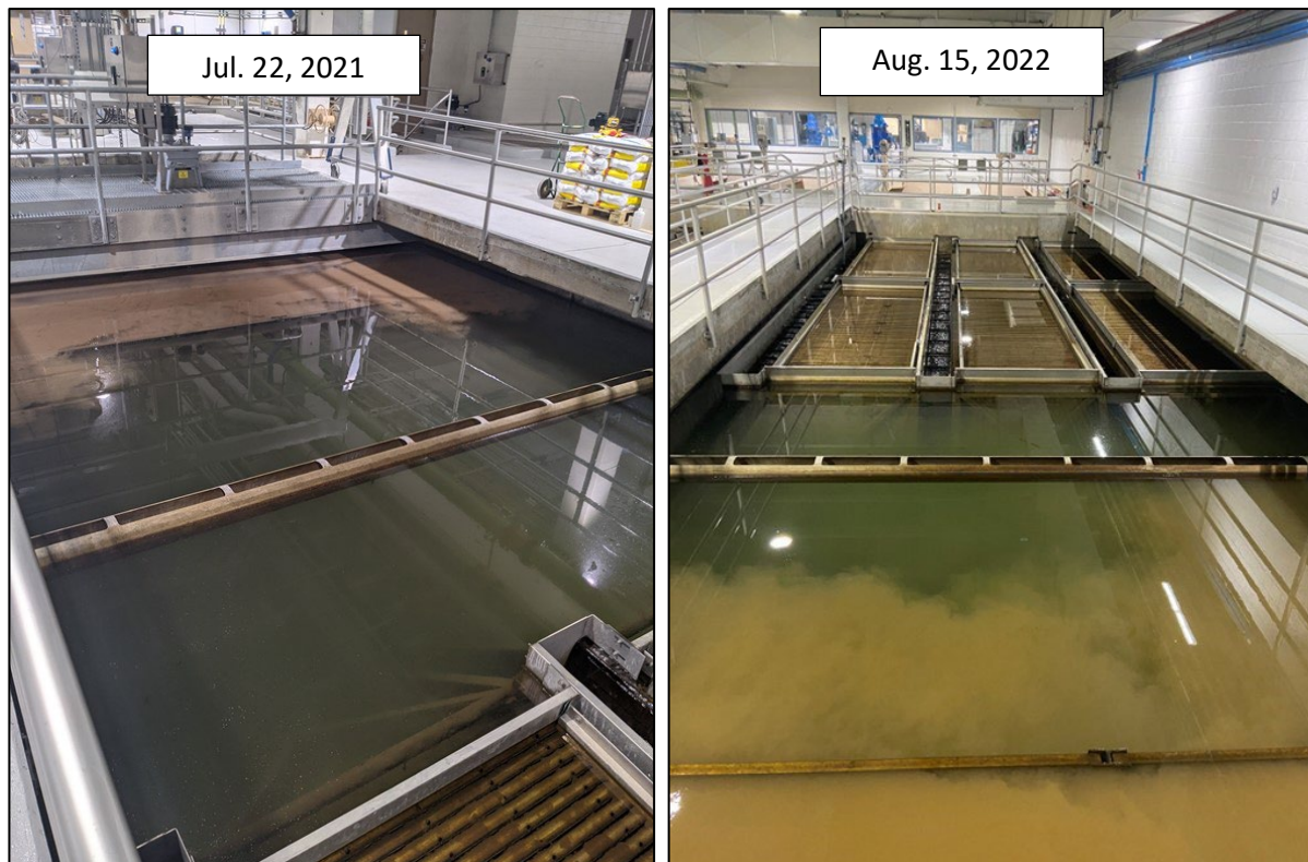
Comparison of ADWF Flocculation/Sedimentation Process during 2021 & 2022 Mudslide Events (note the cloudy, high-turbidity water entering the process was worse in 2022)
