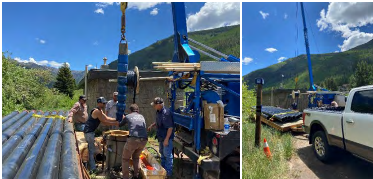
Vail Well R4 Pump and Motor Installation
