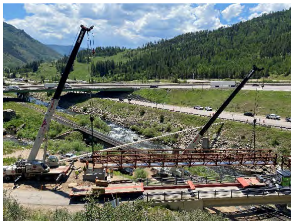
Setting the second bridge segment in place
