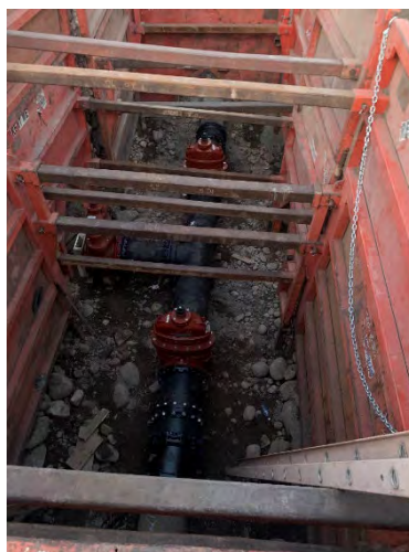
New tee and valve assembly near Edwards DWF
