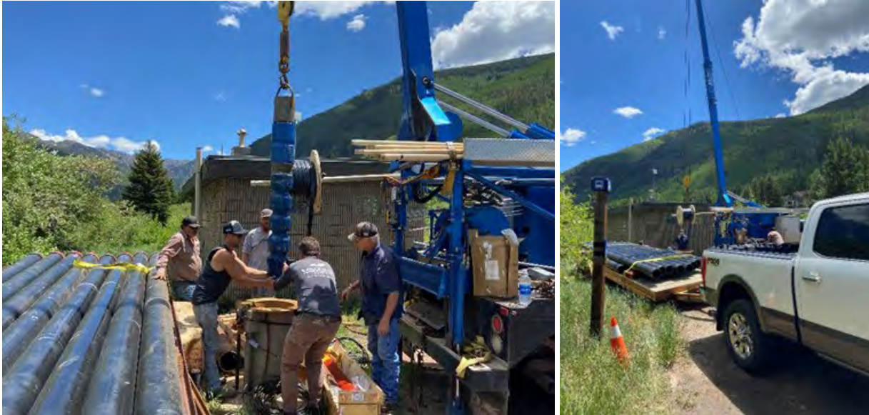
Vail Well R4 Pump and Motor Installation
