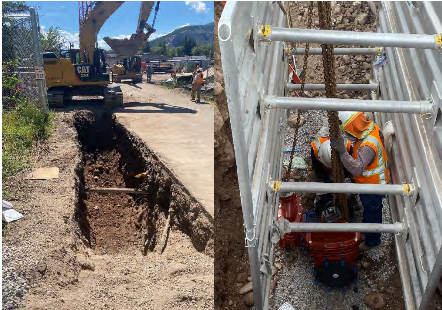
Running pipe through the gate area
