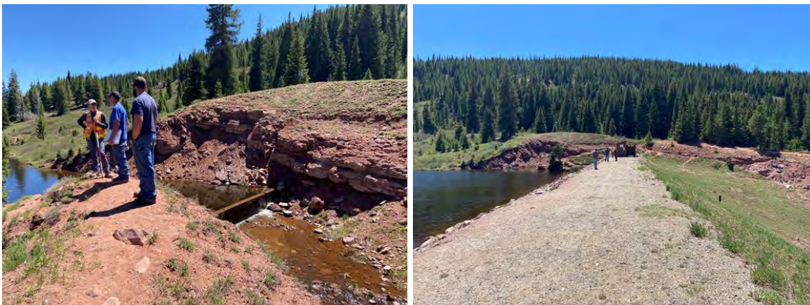
Black Lakes Dam Inspection
