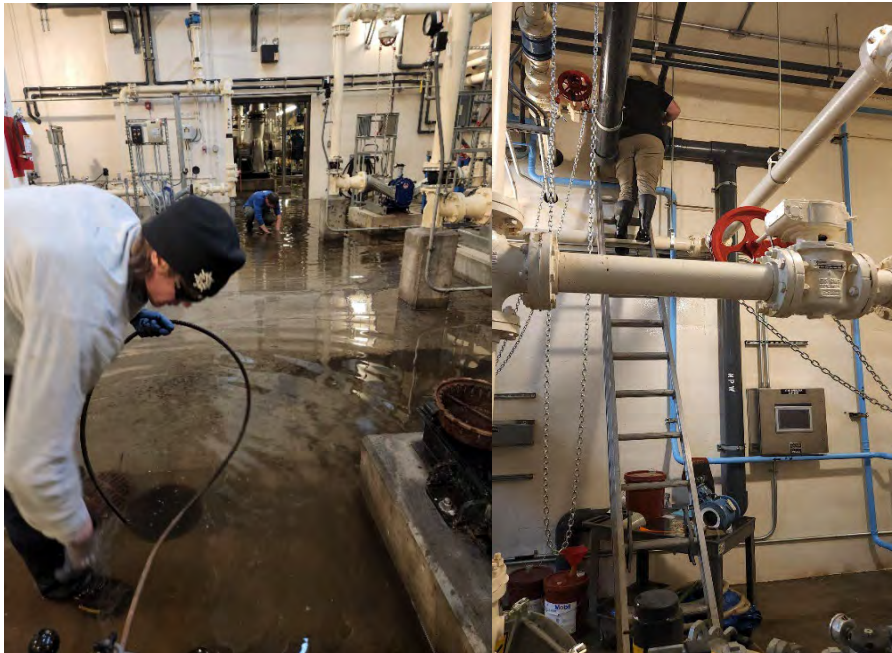
(left) Staff promptly cleaned up standing water in the pump gallery.
