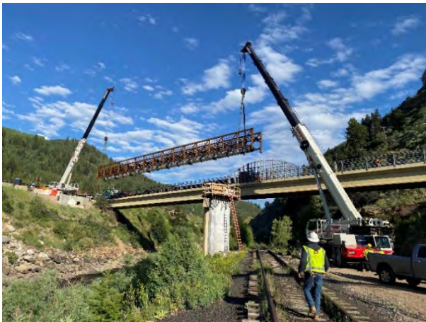
Setting the first bridge segment
