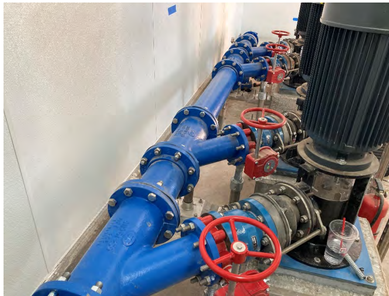
Photo 4: Pump discharge header and piping
