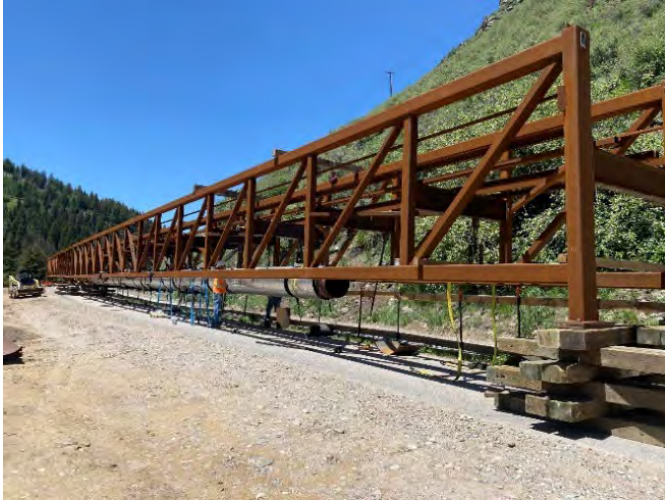
Bridge with pipe installation ongoing
