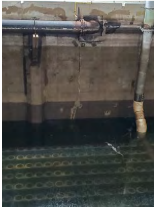
Vail WW aeration basin #4, vertical wall crack evaluation.
