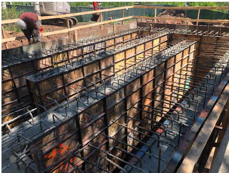
Figure 2: Concrete baffle walls in Clearwell structure
