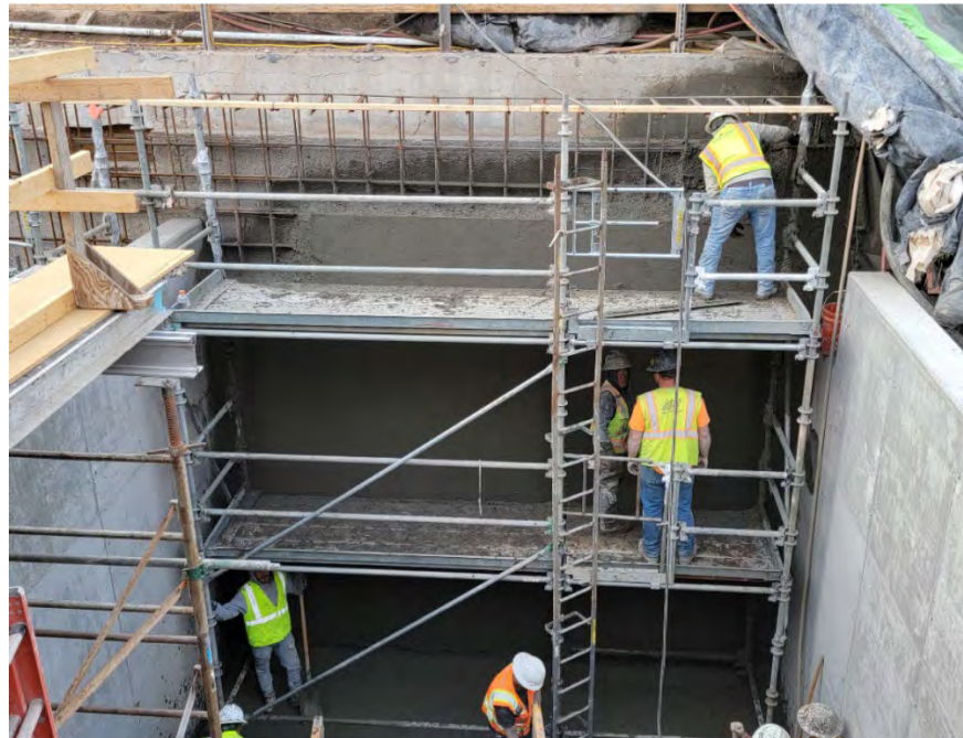
Figure 3. Shotcrete application in aeration basin 1
