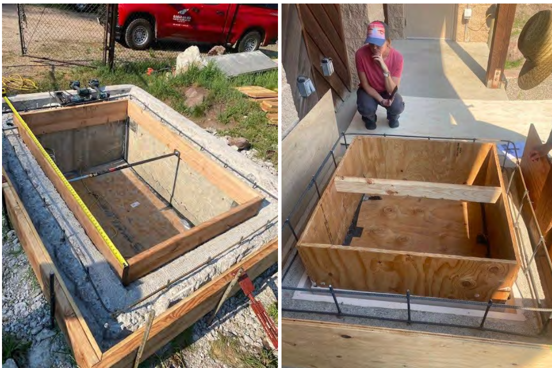
Construction of Water Storage Tank Risers and Hatches (Gore Tank 2 on Left; Gore Valley Drinking Water Facility on Right)
