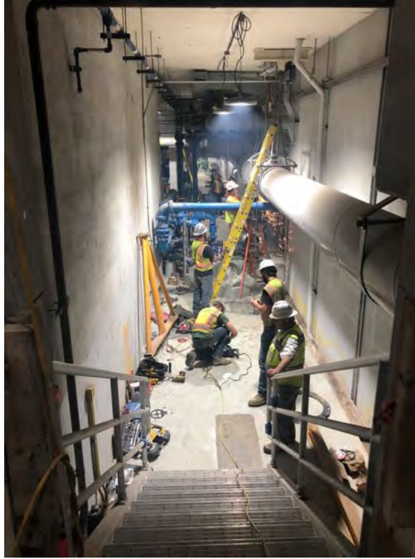
Avon WW aeration secondary clarifier gallery, vertical RAS tie-in procedure.
