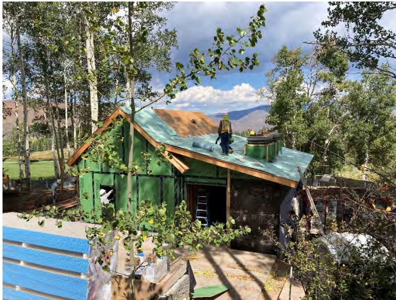
Photo 3: Roofing and Sheathing installation
