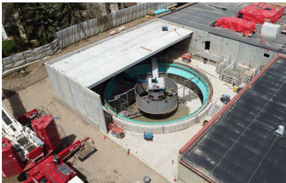
Figure 2: Secondary clarifier and new building construction
