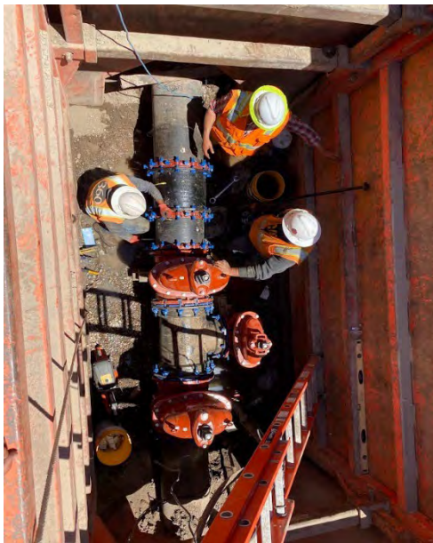
New valve installed
