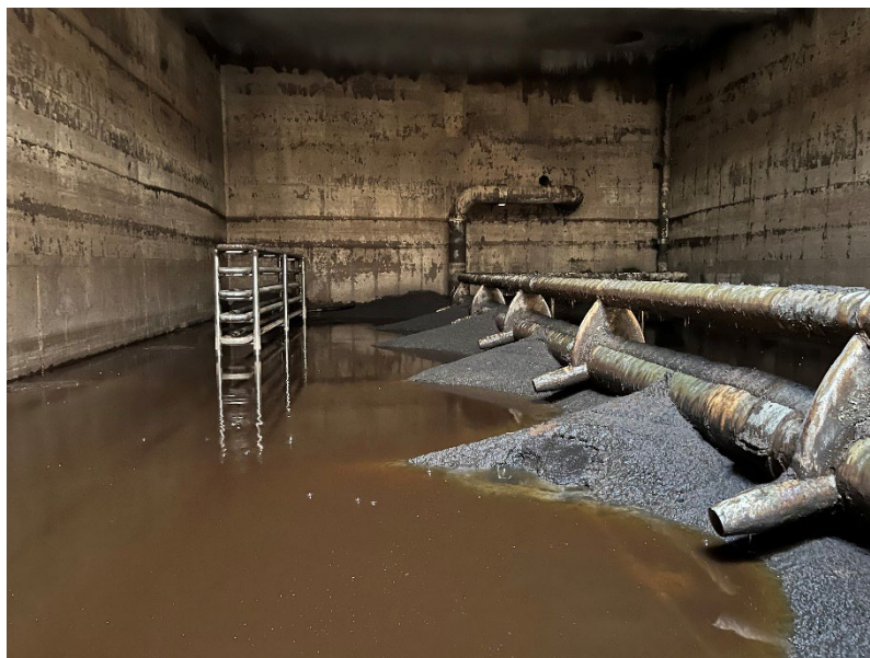
Condition of Edwards WW Final Solids Handling Tank
