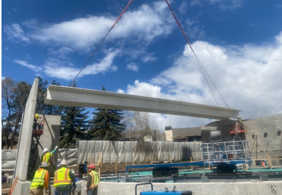
Secondary Clarifier Building Double Tee
