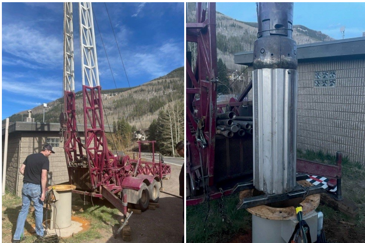
Well R4 Screen Repair on May 11
