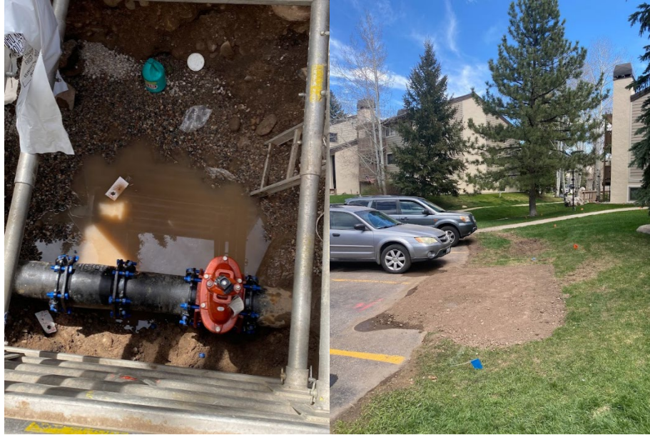
New valve installed
