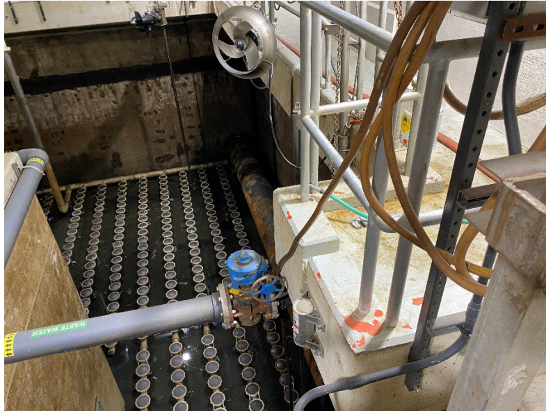
Vail WW Aeration Basin 3. Dewatered for cleaning and inspection
