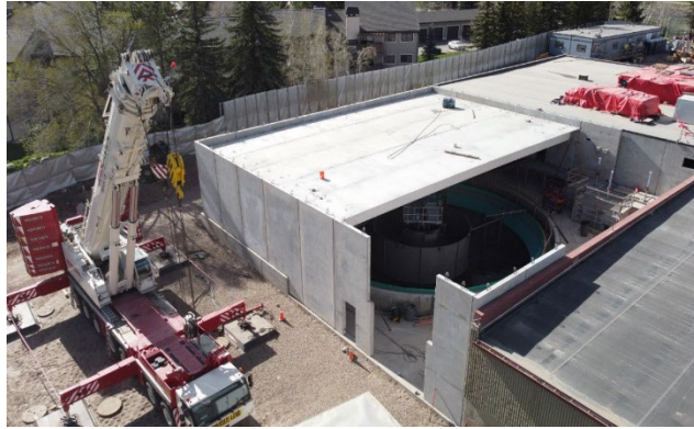
Secondary Clarifier Building Erection
