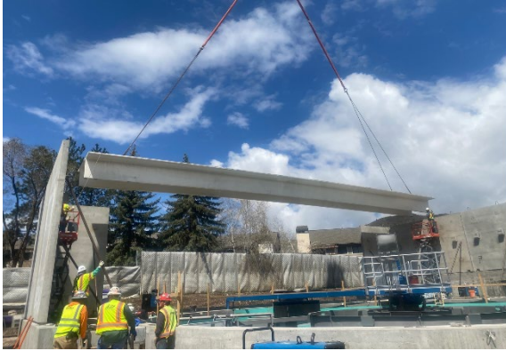
Secondary Clarifier Building Double Tee
