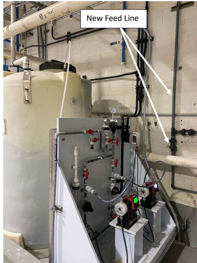
Sodium Permanganate Feed System at ADWF
