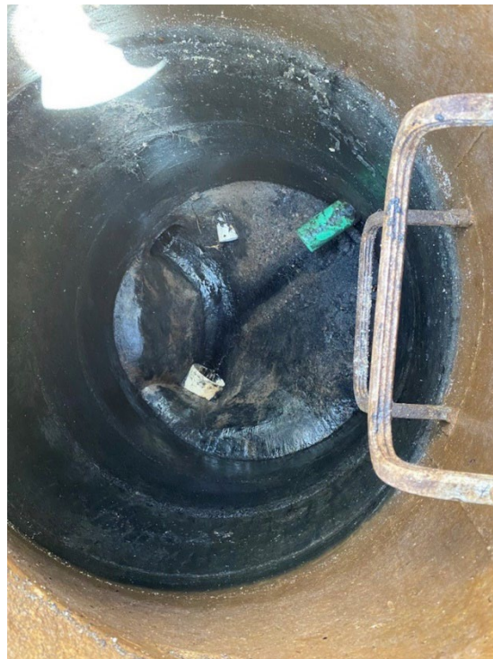
The same manhole after all roots and debris was removed and washed.
