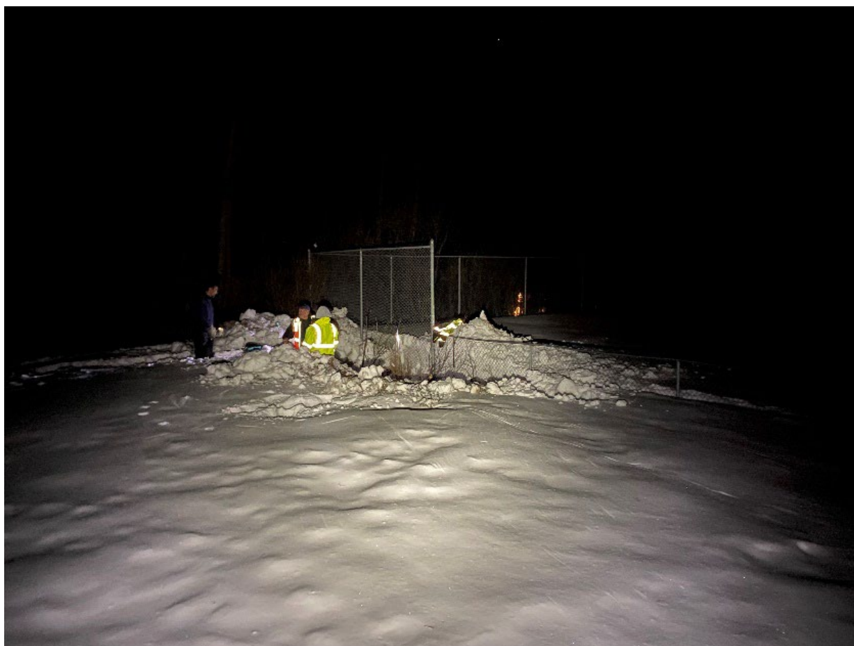
Crew digging through snow to find downstream manhole.
