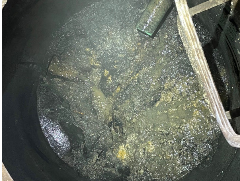
Manhole, after blockage was cleared in pipe downstream.
