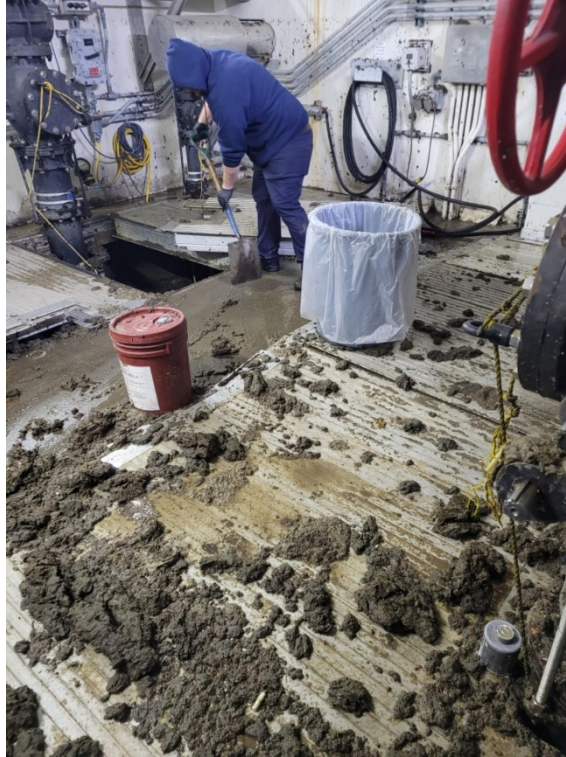
Cleanup of influent pump station began immediately after the sewage had been drained below the floor elevation.
