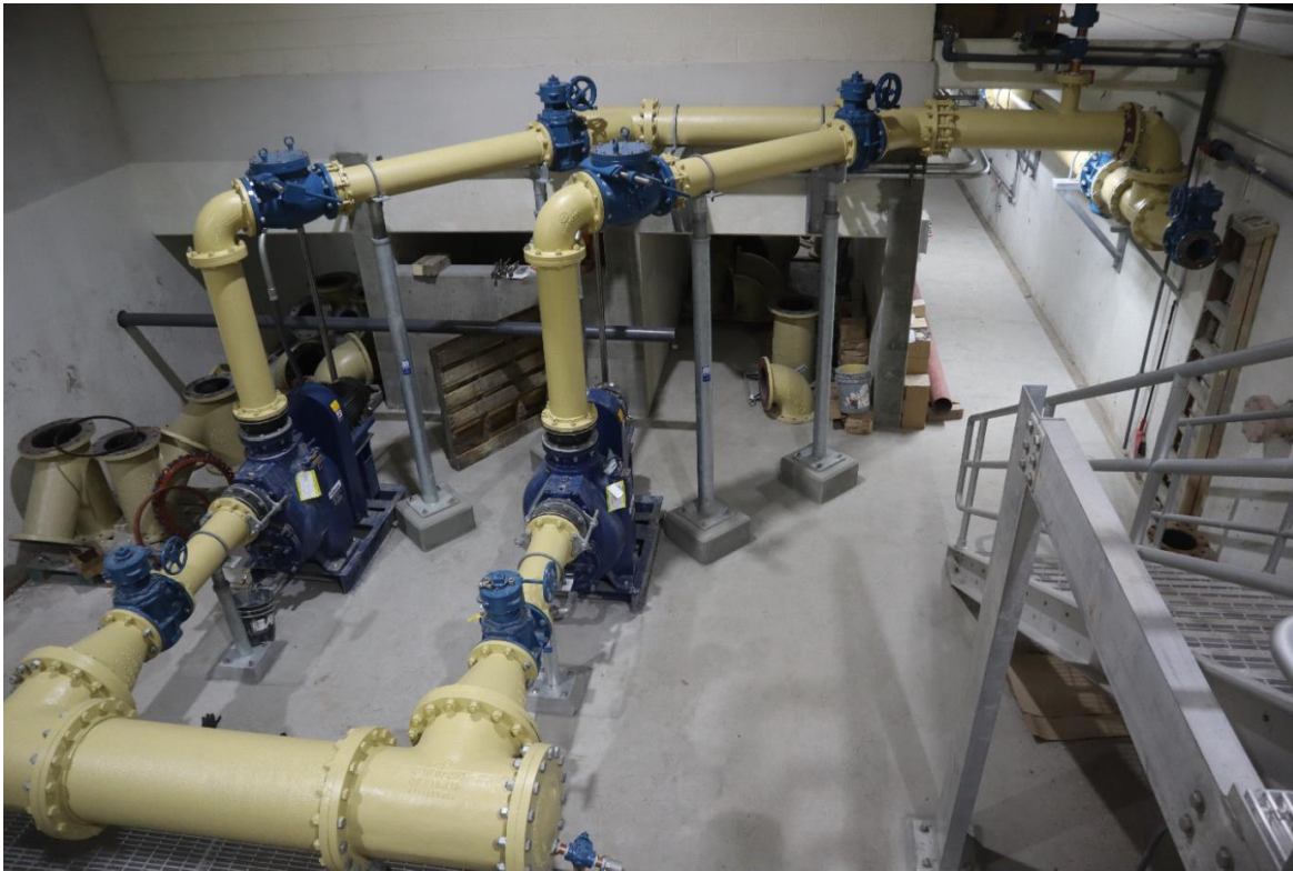
Figure 3. New RAS pumps and piping
