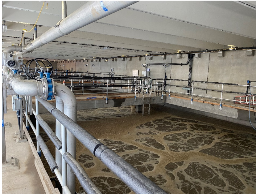
Operation of new Avon WW Aeration Basin #2 secondary process train.
