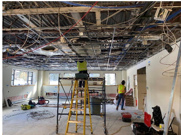
Progress of demolition and electrical rough-in at the new utility services area
