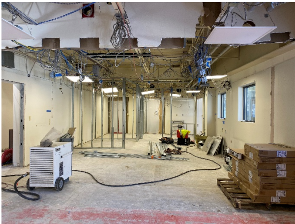
Progress of demo and wall framing in the new customer service area
