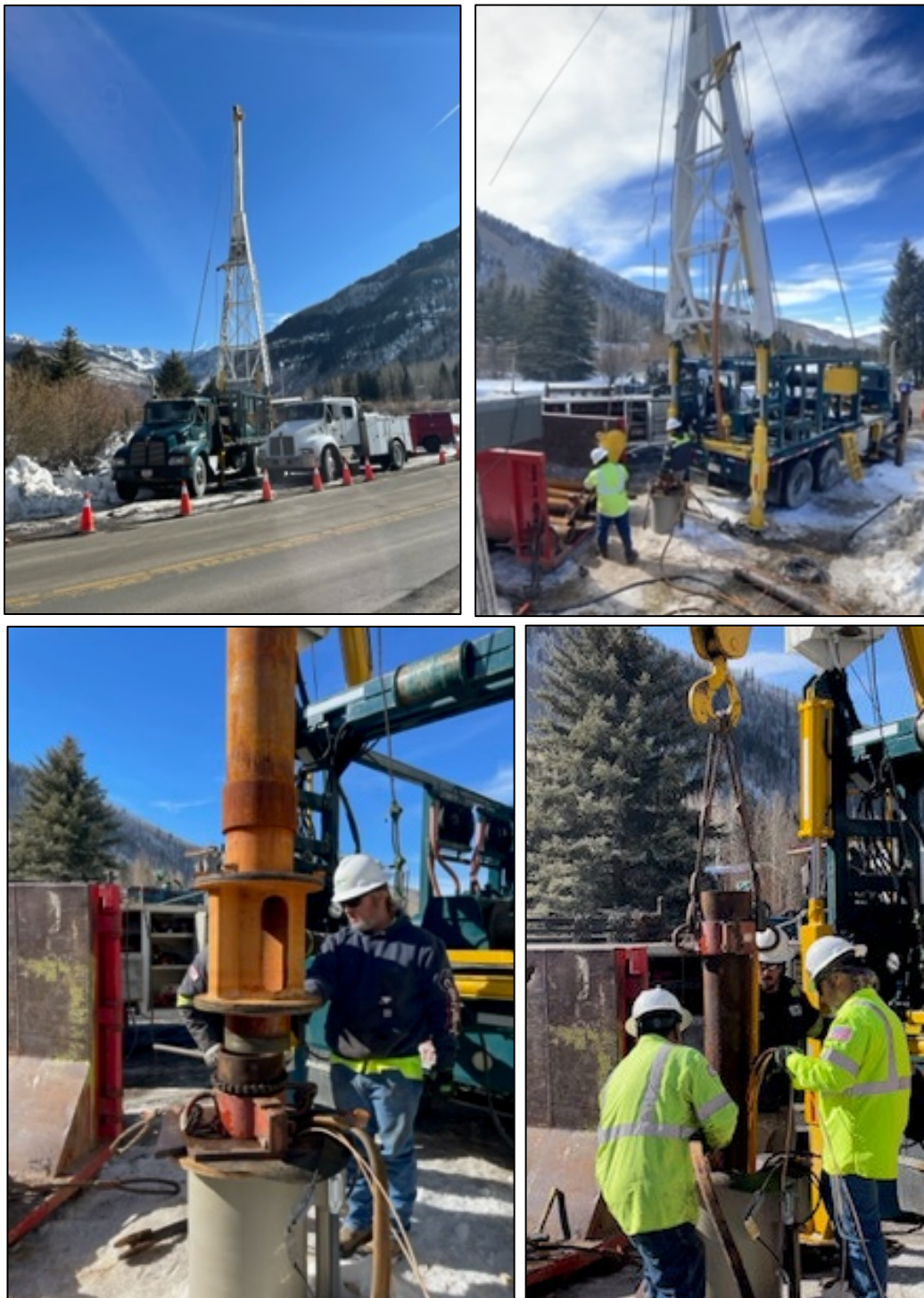
Vail Well R4 Pump and Motor Removal, Feb 15.
