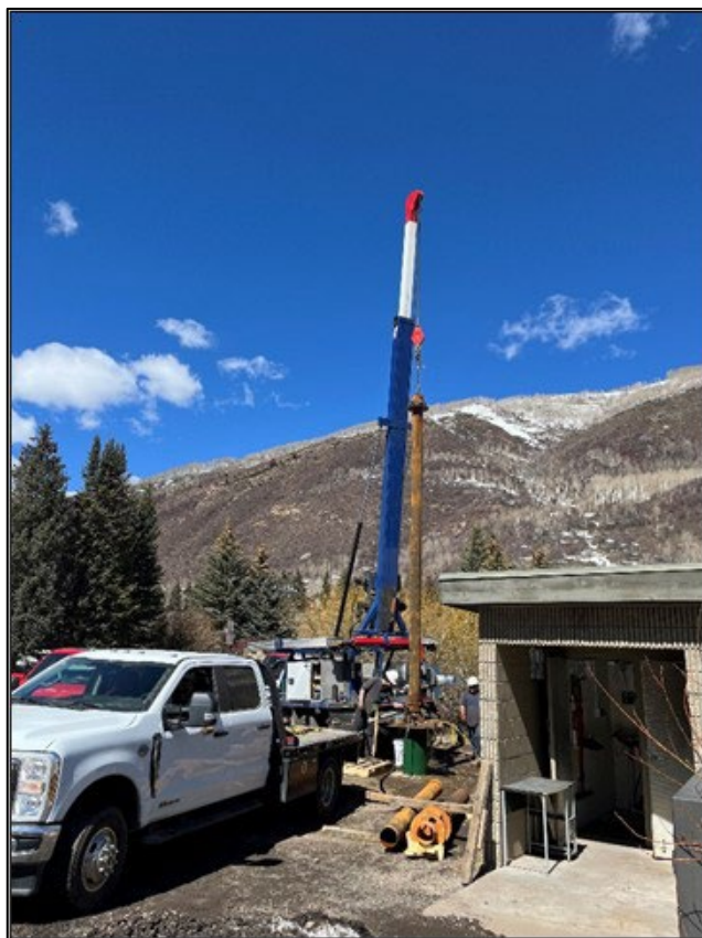
Vail Well R4 Pump & Motor Removal
