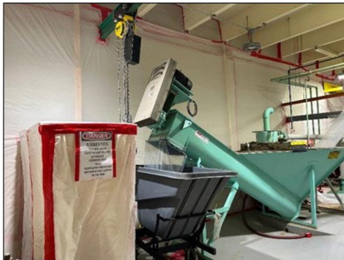
*Asbestos containment barriers installed in VWW headworks*
