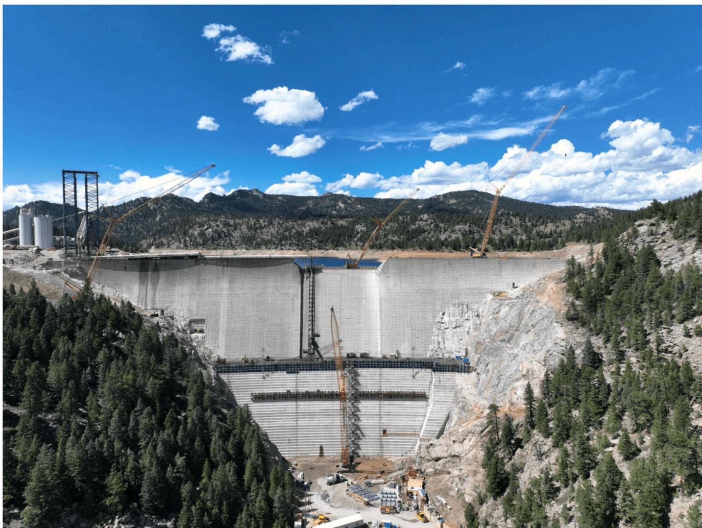
The stair-step reinforcement and raising of Gross Reservoir Dam in Boulder County, now well underway. The project is the key to Denver Water's massive expansion of the pool at Gross Reservoir, which prompted years of negotiations with Boulder County and environmental groups on mitigating impacts on surrounding land and watersheds. (Source: Denver Water)
