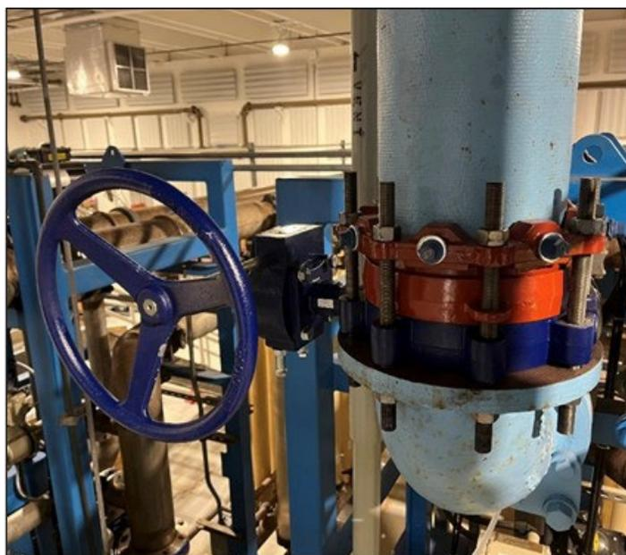
*EDWF membrane system “block-and-bleed” valve installation*
